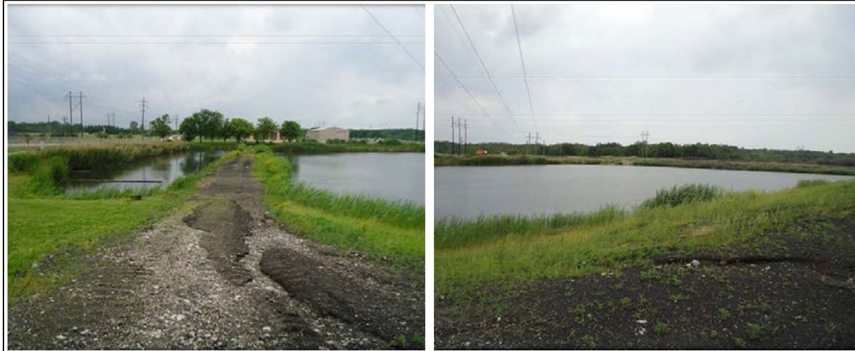
Figure 3.2 2011 Photographs of Pond 4 – General Conditions. Source: Kleinfelder, 2013.
